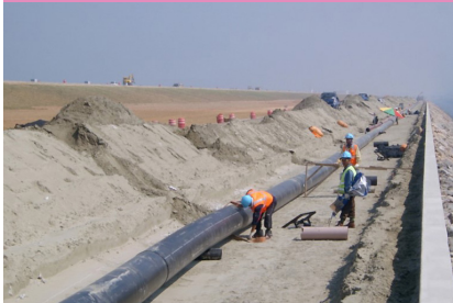
Saemangeum, Korea Water Supply Pipe Project
