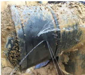
Identification of precise location of Underground Pipe.
