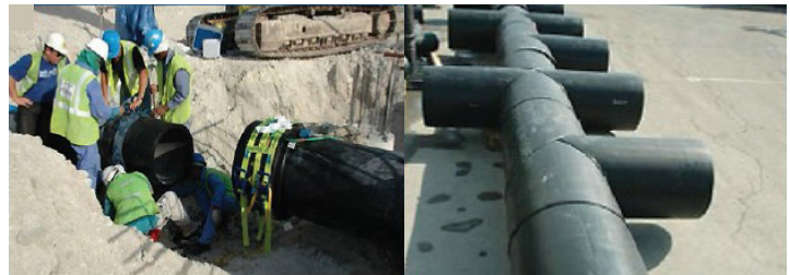
Dubai Palm Island Project Electro Fusion
