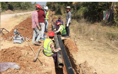
Myanmar, Monywa Water Supply Project
