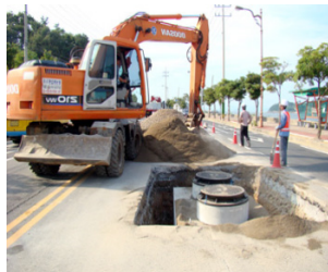
Avoid unnecessary digging. Saves unnecessary street blockage and labor
