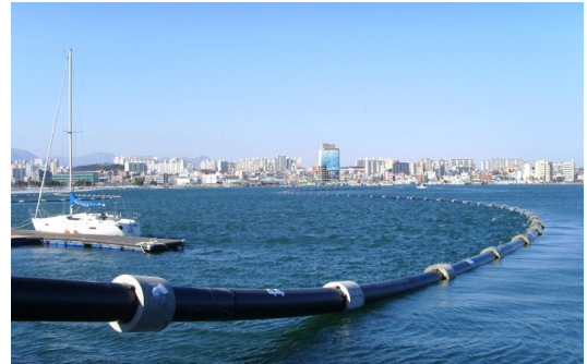
Sokcho, Korea Deep Ocean Water Intake Pipe Project
